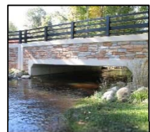
Figure 4: Three-sided box bridge
