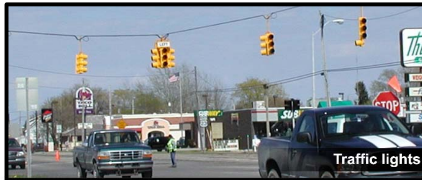
Figure D-1: Example of traffic signals
